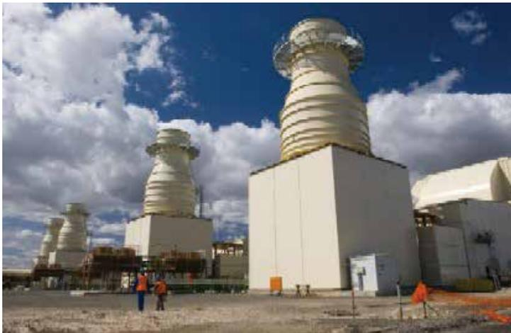
*Ankerlig Power Station in the Western Cape. Eskom is being forced to run this station for 17 hours a day – well above its design capacity of 3 hours a day.*
