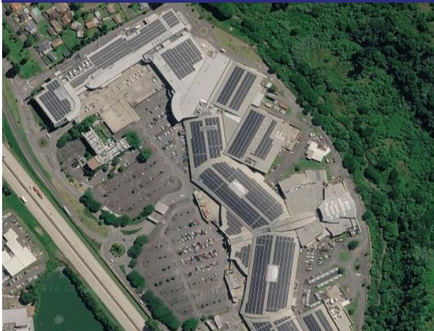
Liberty Midlands Mall has one of the largest rooftop solar plants in South Africa at 6.5MWp, reducing the mall's reliance on electricity from the grid by 36%
